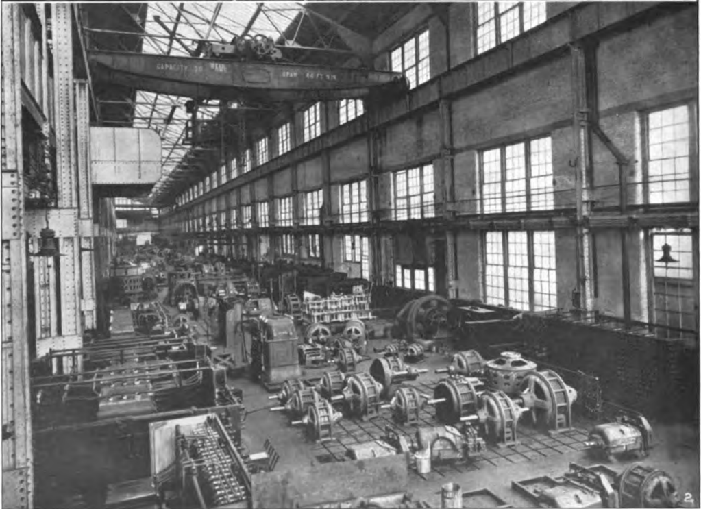
Departments (1) No. 18; (2) No. 60, Works of General Electric Company, Schenectady, N. Y.
